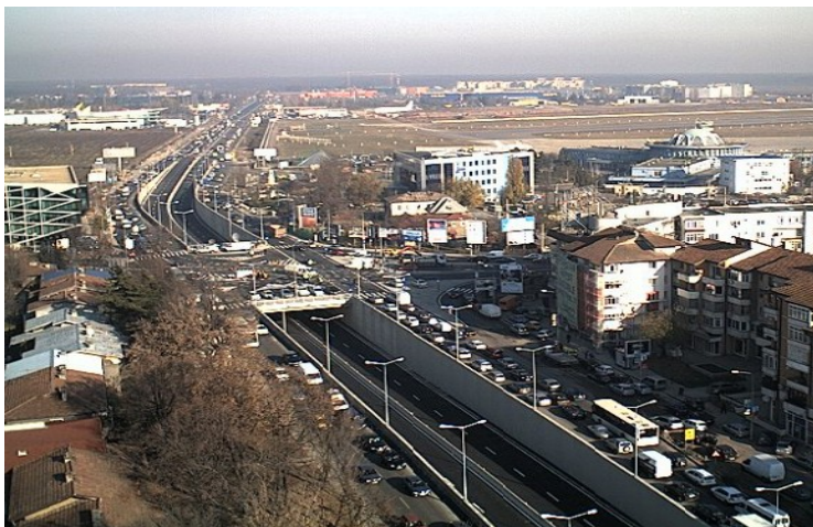
PASAJUL BANEASA, antreprenor general fiind firma portugheza LENA CONSTRUCTII
